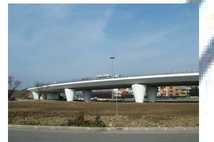
Figure 4: viaduct Langhirano Highway.
